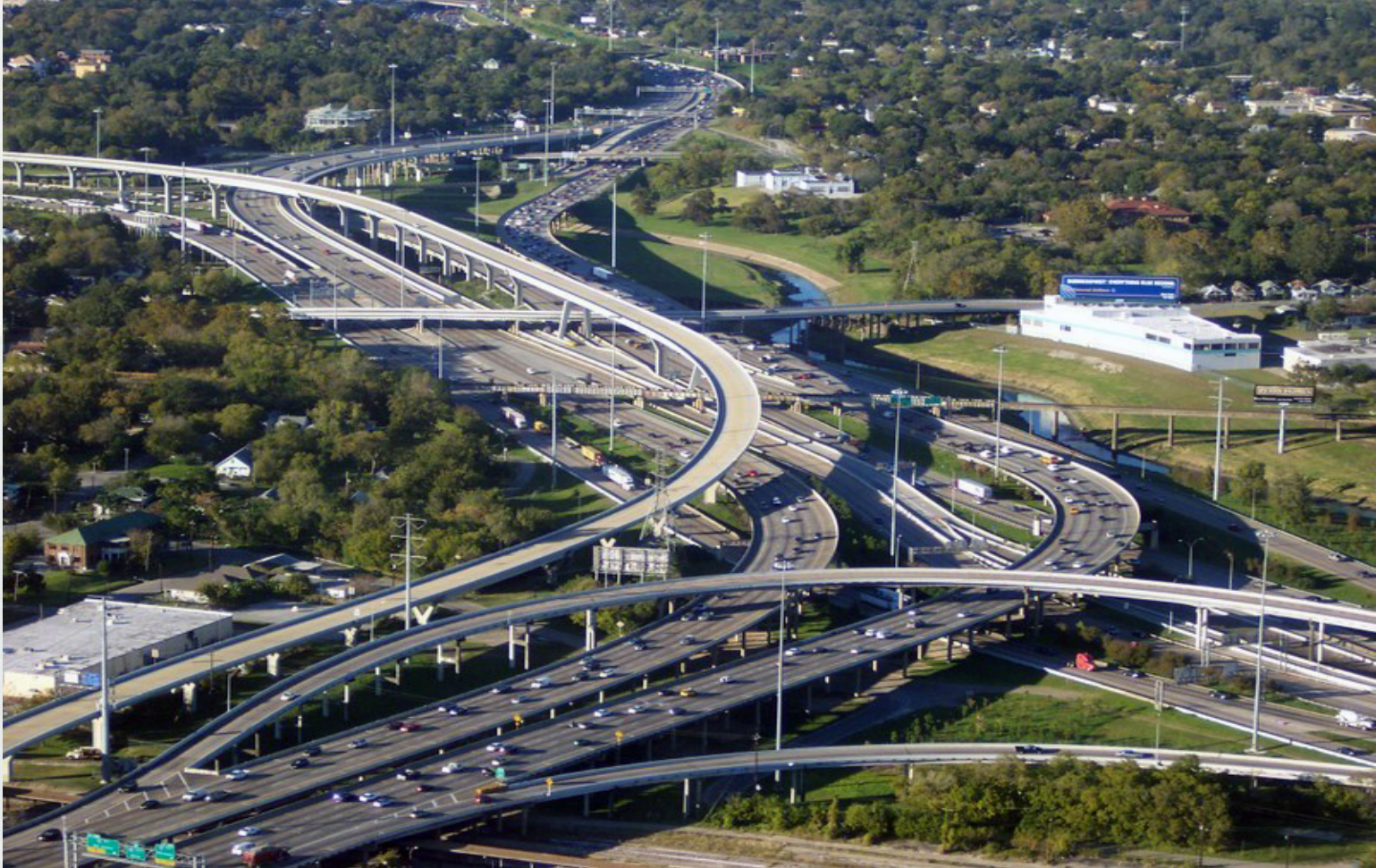
I-10 and I-45 interchange northwest of downtown Houston.
