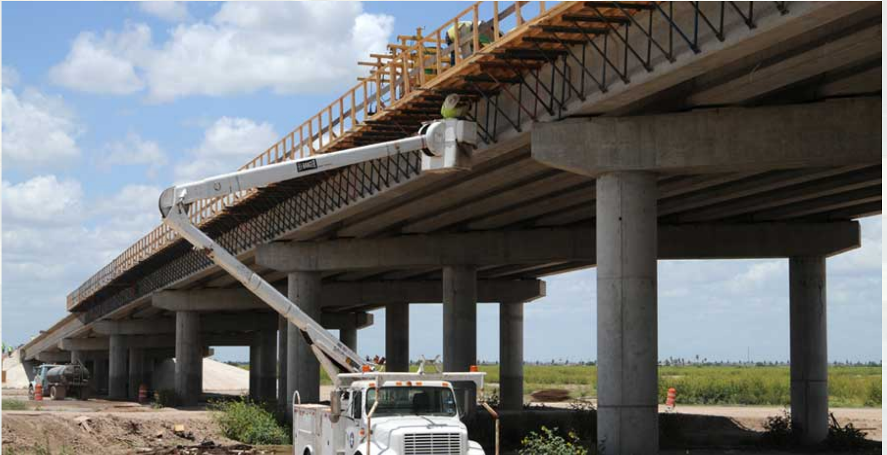
Anzalduas Bridge Construction, McAllen, Texas
